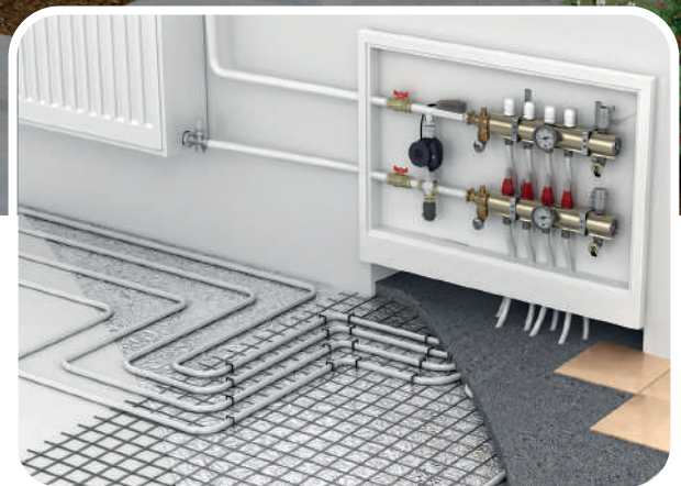
Suelo radiante / Underfloor heating
